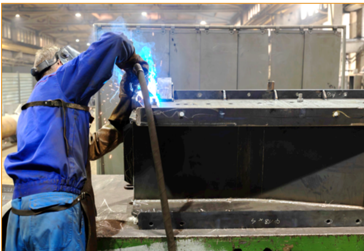
Fig. 2 One stage in manufacturing a load-bearing steel structure cut component.
